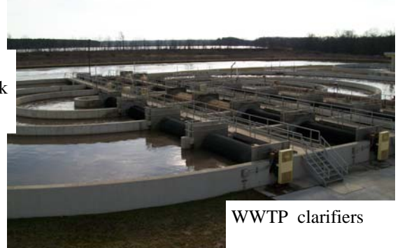
WWTP photo of the clarifiers and aerator
